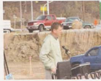
Jason Stephens, Lawrence County Commissioner is seen here at the groundbreaking of the South Point Comfort Suites in November.
